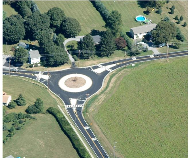
The roundabout at the intersection of Route 82 and Doe Run in East Marlborough Township is an example of a safety and circulation improvement appropriately scaled to the surrounding context.
